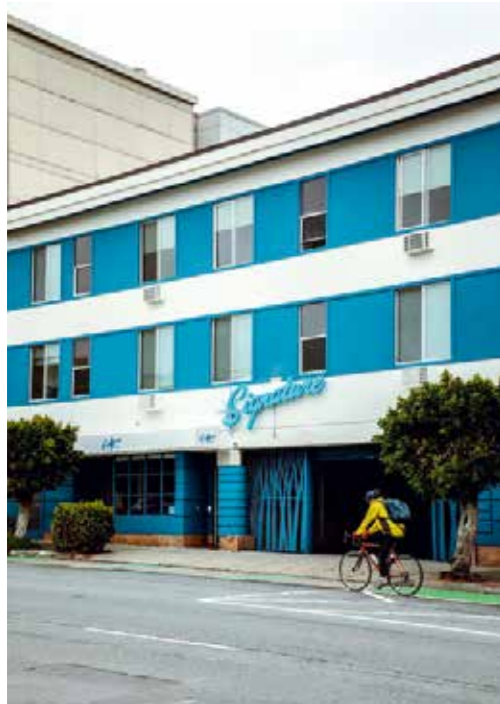
From top The motel's striking cyan façade stands out amid its surroundings; rooms at Signature San Francisco are inspired by Mid-Century Modern design
